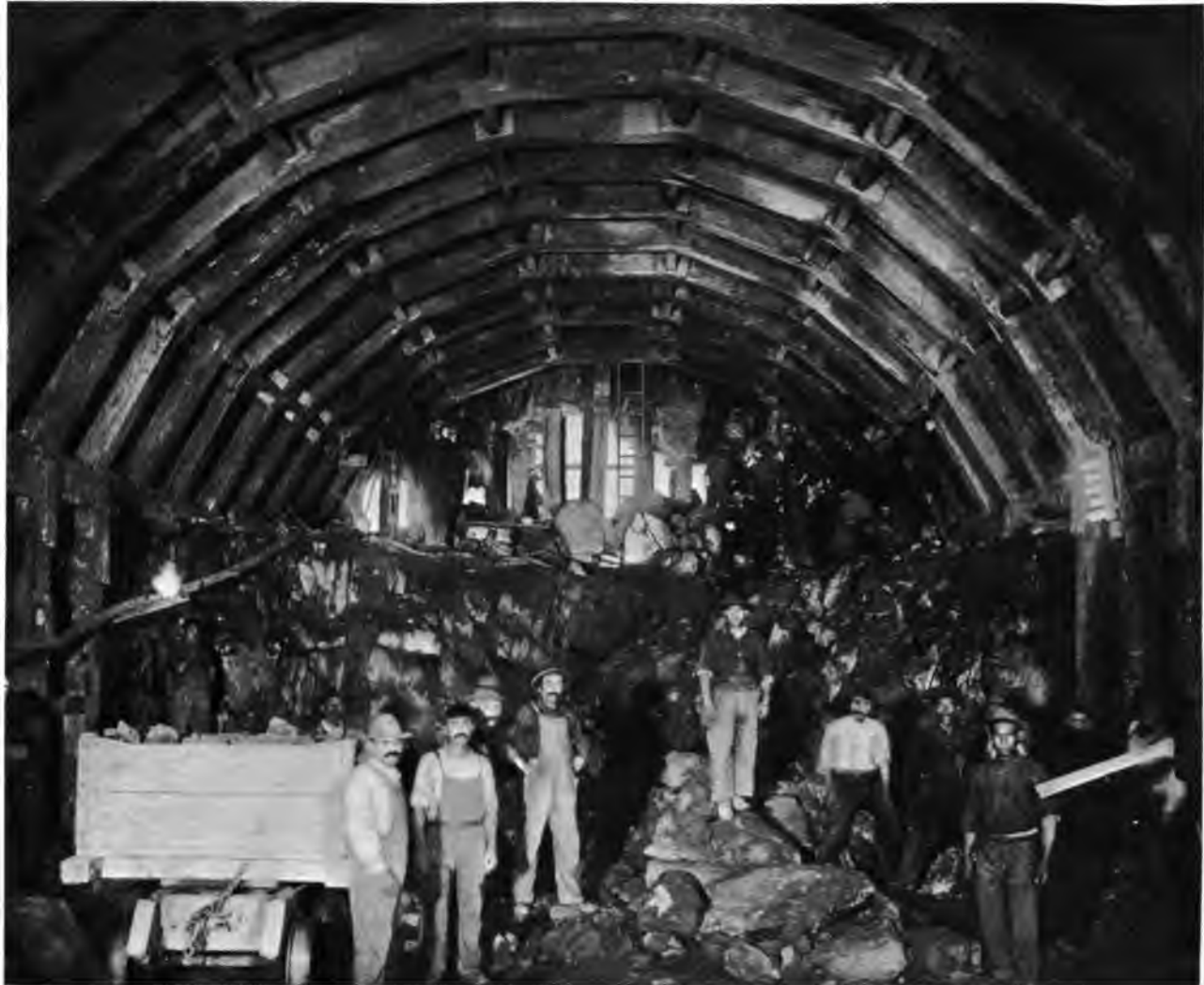
CONSTRUCTION OF FORT GEORGE TUNNEL
